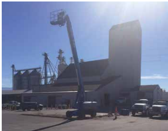
Demolition of the old Agronomy North plant.
