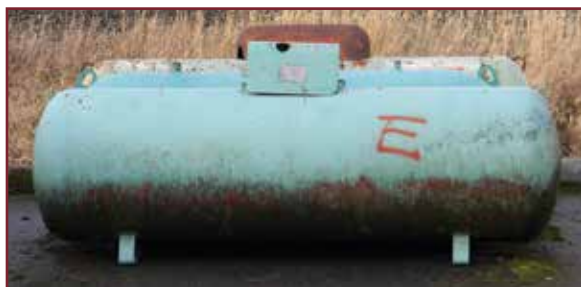
A circa 1967 tank before blasting and repainting.
