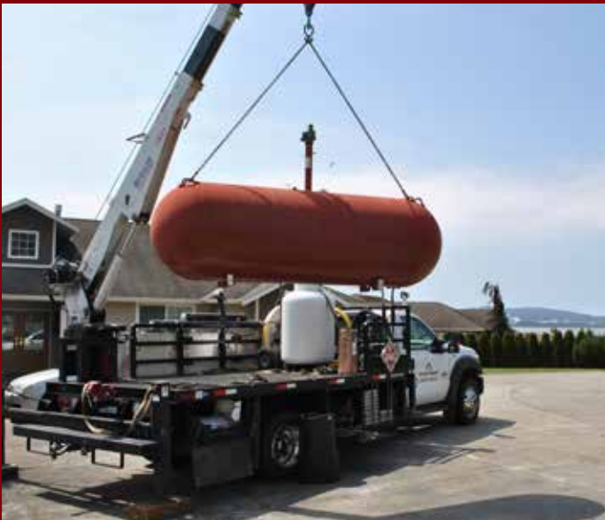
Setting an LP tank on Whidbey Island.
